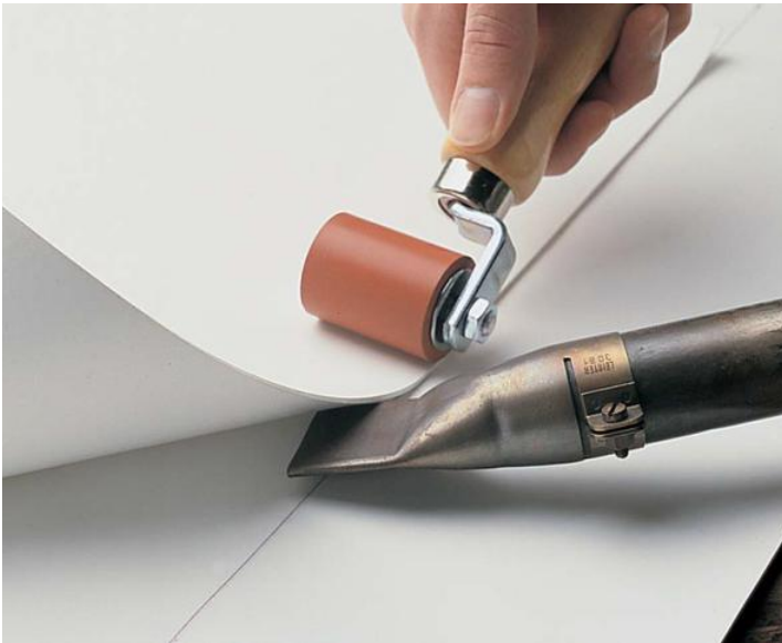
Flex single ply membranes are hot-air welded and provide seams as strong as the material itself. Flex membranes stay repairable indefinitely.
