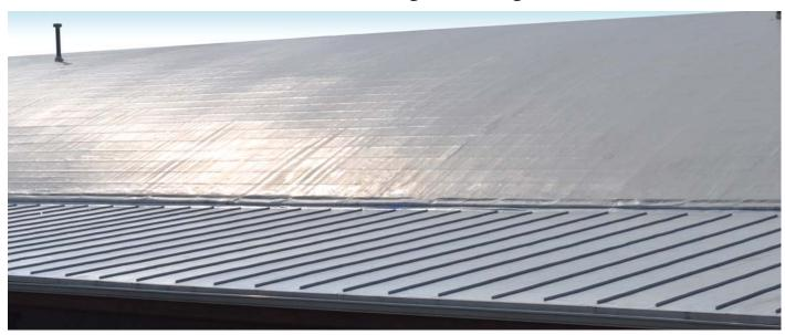
The Flex PVC Roof Rib Profile is designed specifically as a high quality, low cost alternative to the standing seam metal roof. The Roof Rib duplicates the look of a traditional standing seam, while saving the building owner the long term maintenance costs of a metal roof. The Flex PVC Roof Rib Profile is manufactured from the same Flex compound as the Flex Roof membranes and is available in a wide range of colors to meet the requirements of any building design
