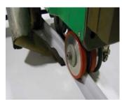
hot air welded into place preventing punctures to the membrane and ensuring a secure, watertight installation. The versatility of the rib allows for unlimited flexibility in the spacing and layout.
