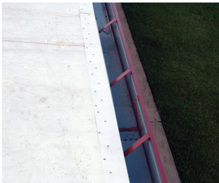
FlexClad™ metal drip edge, properly secured
