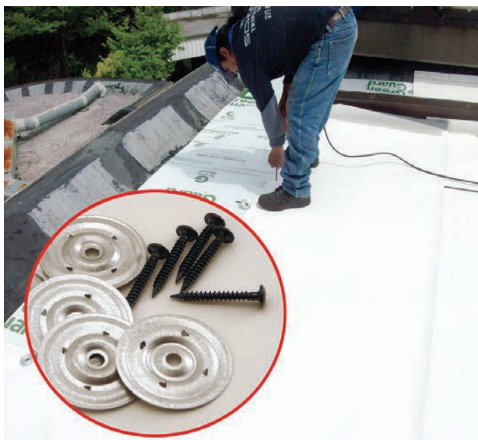
Flex fasteners and screws help make installation easier and faster.
