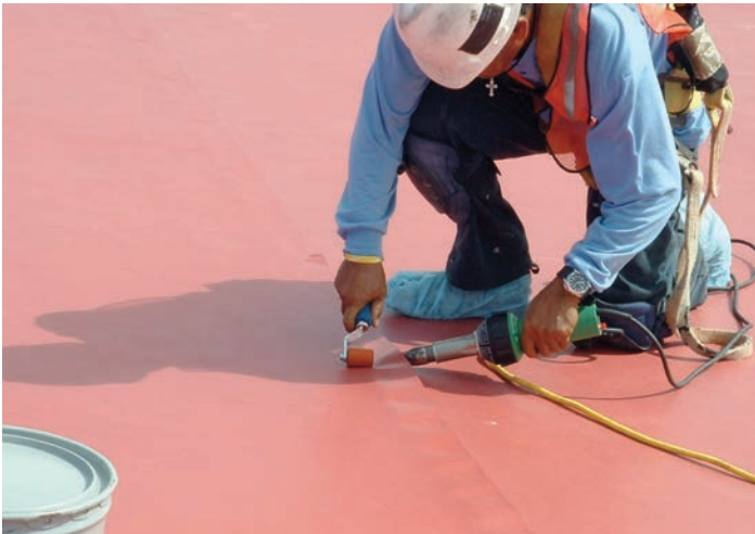
Hot air welding with a hand held tool
