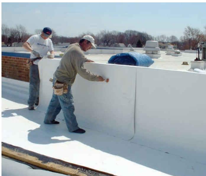
Rolling wall flashing into place
