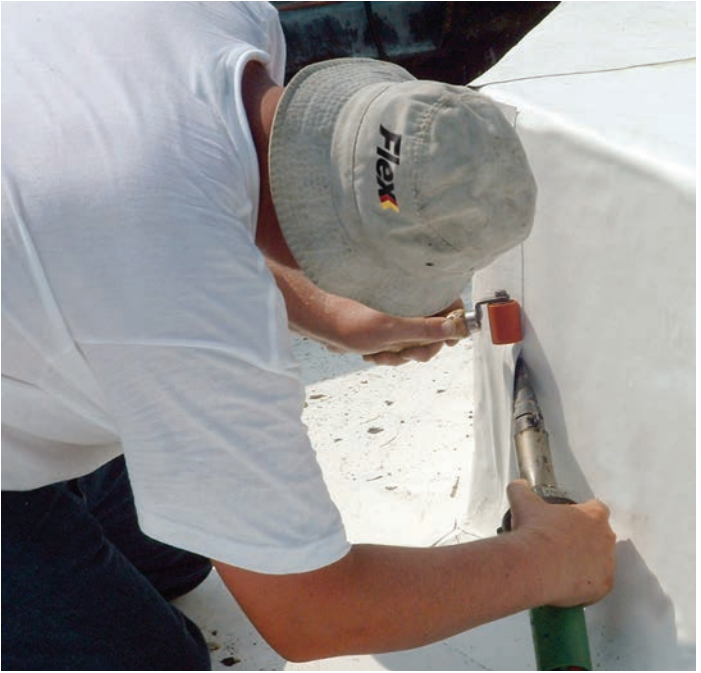
Using a hand held hot air welder to install wall flashing
