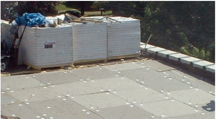
Mechanically fastened Flex insulation board
