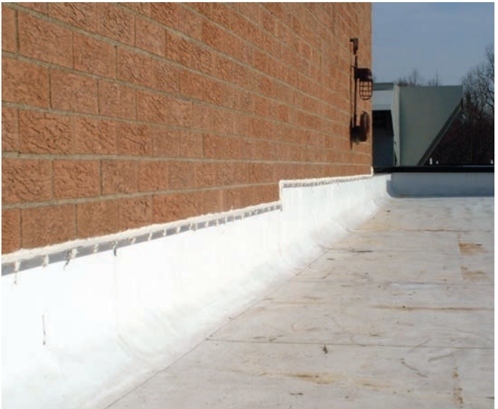
Wall flashing with Flex Lip-T bar, with approved caulking
