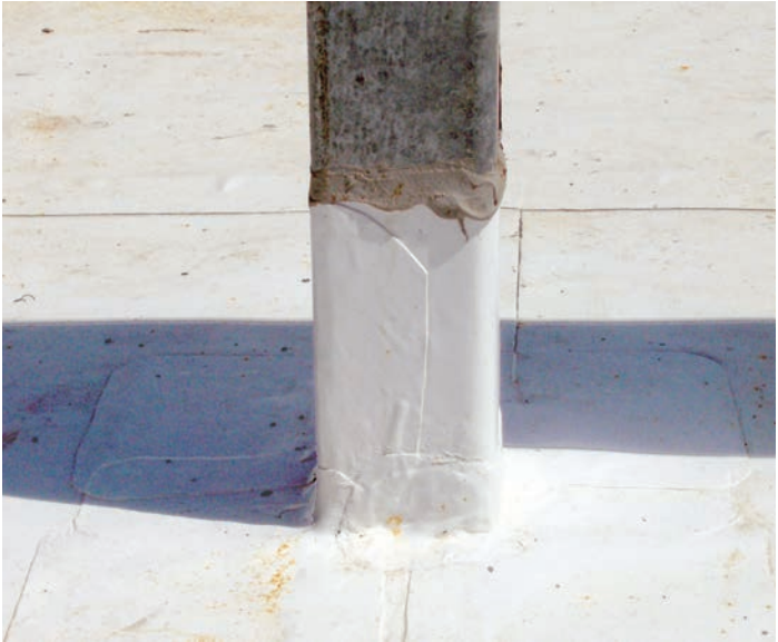
Post support flashing, available pre-formed from Flex
