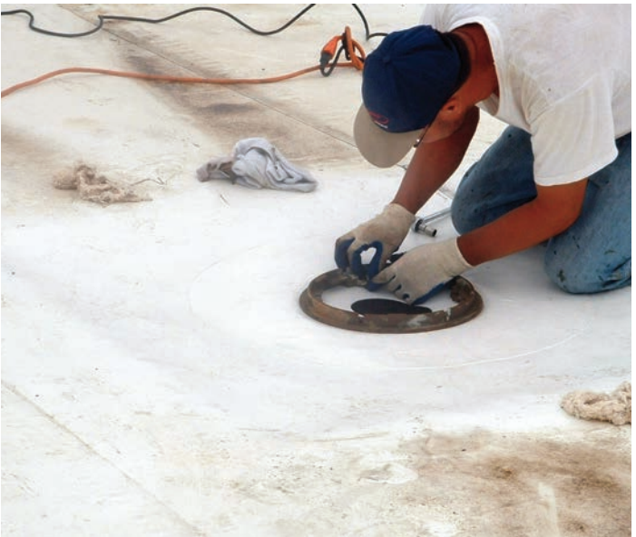
Tightening the clamping ring on a drain flashing
