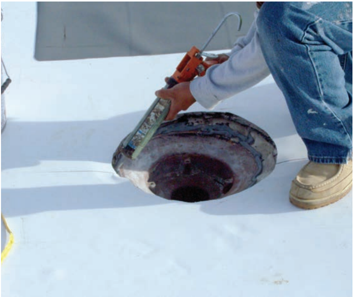
Applying water block to a drain flange under the field membrane
