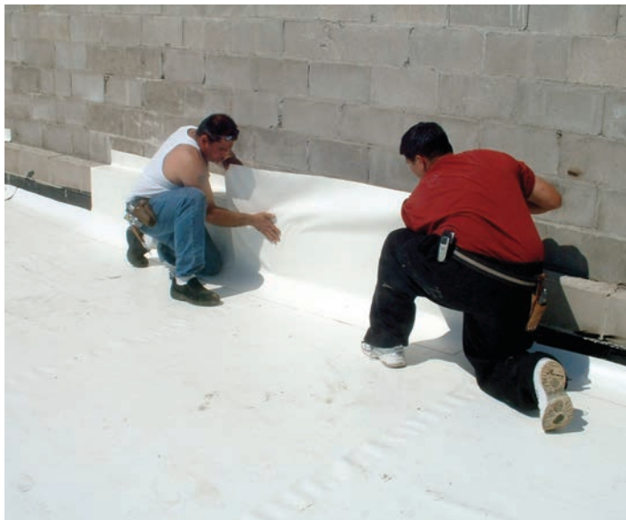
Hanging the wall flashing
