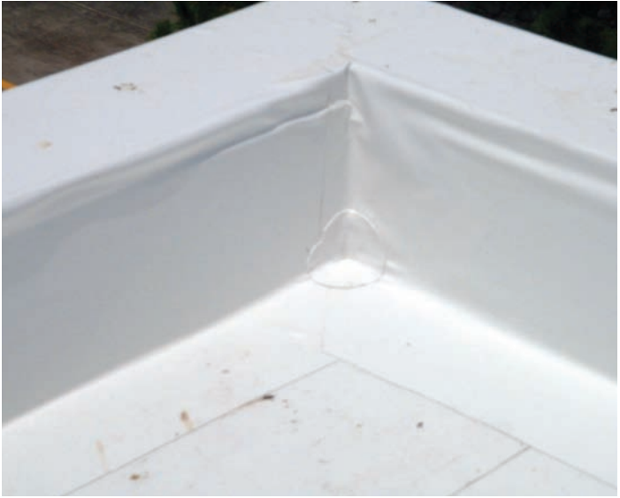
Pre-formed inside corner flashing
