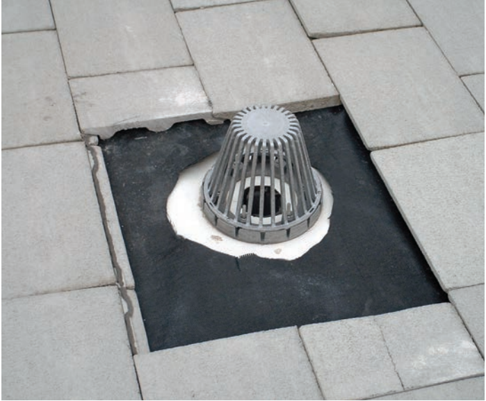
Pavers installed over properly flashed drain detail
