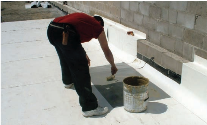
Applying flashing adhesive
