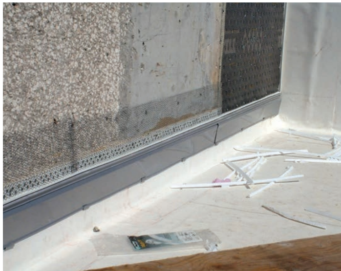
Wall flashing with metal counter-flashing
