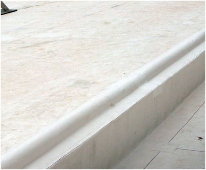
Expansion joint cover, with Flex TPO Reinforced Flashing Membrane
