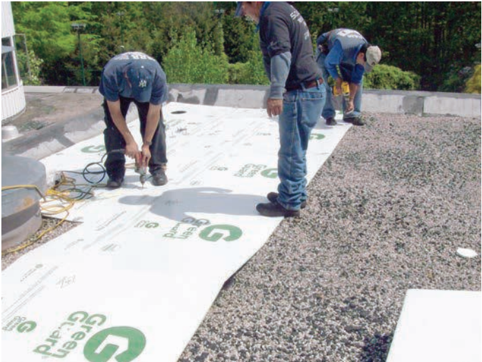
Placing Flex fan-fold GreenGuard re-cover board
