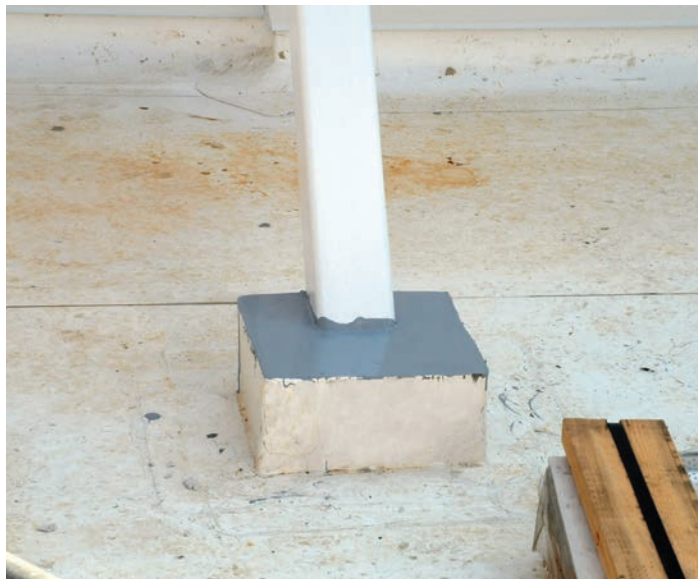
Pitch pan topped off with Flex Pourable Sealer
