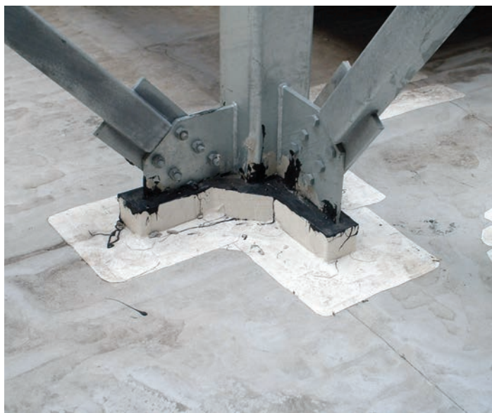
Pitch pans solve difficult flashing details
