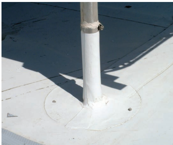
Flex Split Pipe Boot, a pre-fabricated flashing
