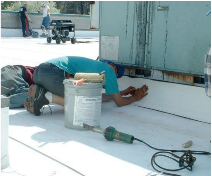
Flashing existing mechanical unit
