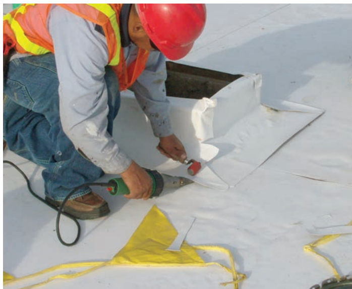
Hand welding a field-fabricated flashing
