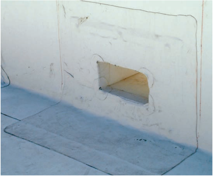
Through-wall scupper made of FlexClad™ Metal
