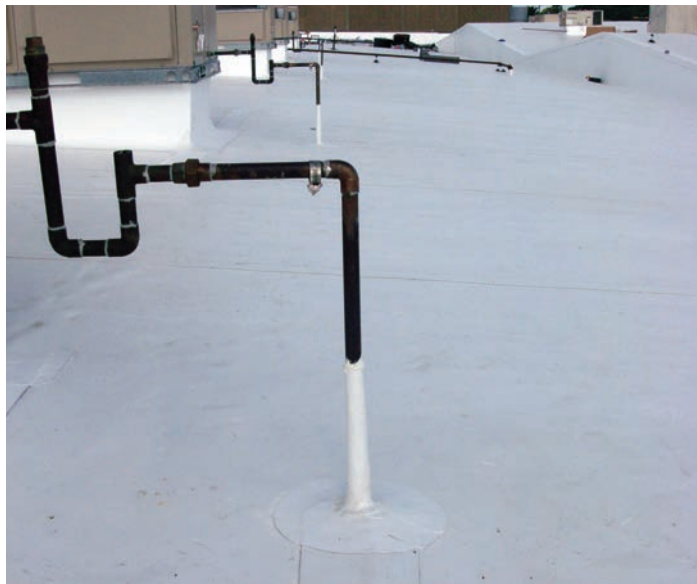
Field-fabricated method with Flex TPO Flashing Membrane
