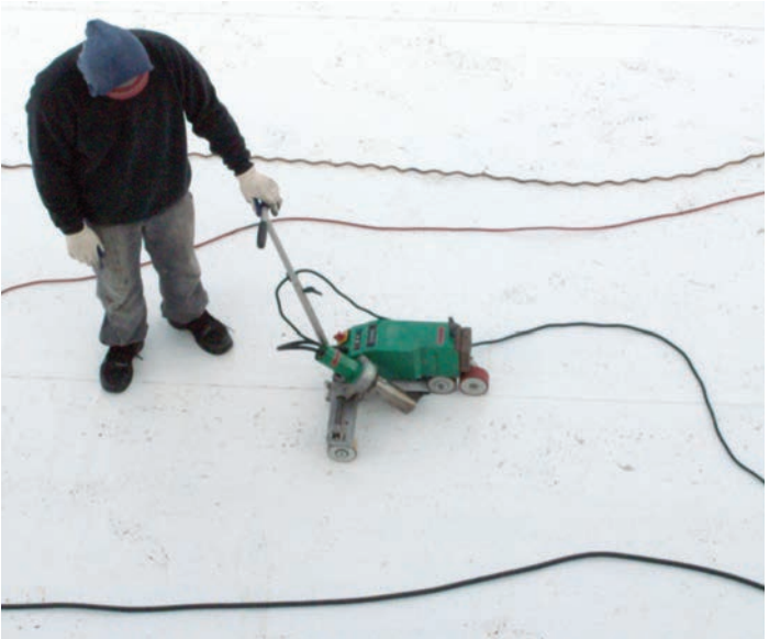
Automatic hot air welder allows workers to operate upright, which is more comfortable and much faster.
