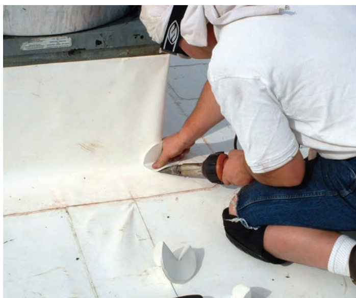
Hand welding a pre-formed outside corner flashing
