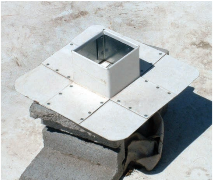
FlexClad™ metal pitch pan, fabricated by the contractor
